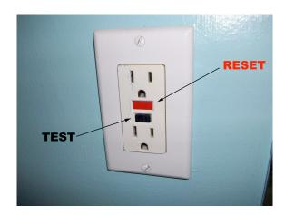
The normal position is that the **RESET** (or RED) button is PRESSED IN and the **TEST** (or BLACK) button is OUT. If the GFI trips, then the **RESET** button will POP OUT. Normally you can just reset the GFI by (a) making sure that the circuit breaker is ON, and (b) pressing the **RESET** button IN. If it will NOT stay in and it immediately pops back out there is a current leak (contact an electrician).
